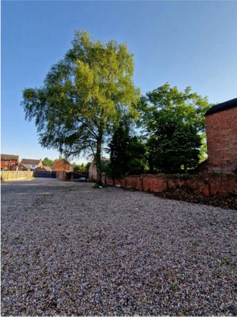
Wall looking to the rear.
